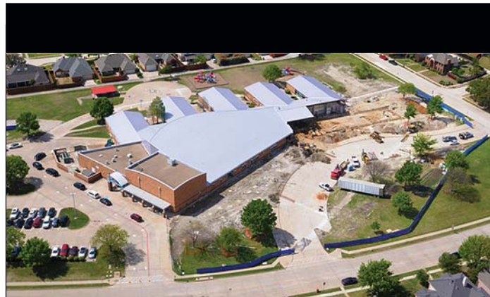
Cadence McShane has been selected by Plano Independent School District to serve as Construction Manager At-Risk for the construction and renovation assignments at Bethany and Hedgcoxe Elementary Schools in Plano, Texas, totaling 154,623 square feet.
